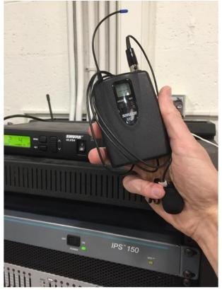
Or, if they have a XLR connector on their microphone they can plug in to the system's sound by unplugging the cable at the rear of the Shure system.
